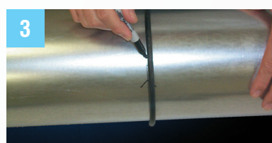
3 Use provided O-ring to mark for cut.
