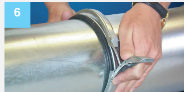
6 Place QF Clamp over the O-ring and end of Quick-Fit Sleeve.
