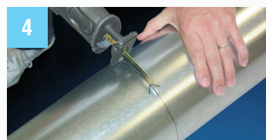
4 Drill access hole, then cut Pipe with saw.
