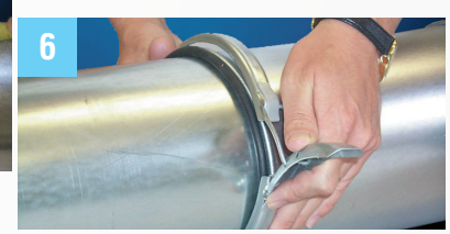
6 Snap QF Clamp over O-ring and one end of Quick-Fit Sleeve.
